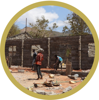
ICT Lab Construction Mlugh Primary School
